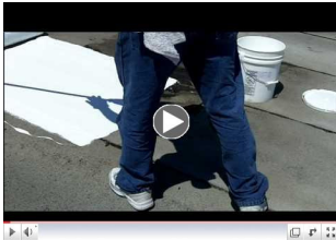
Roof Repair YouTube Video
