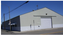
SureCoat Metal Roofs
